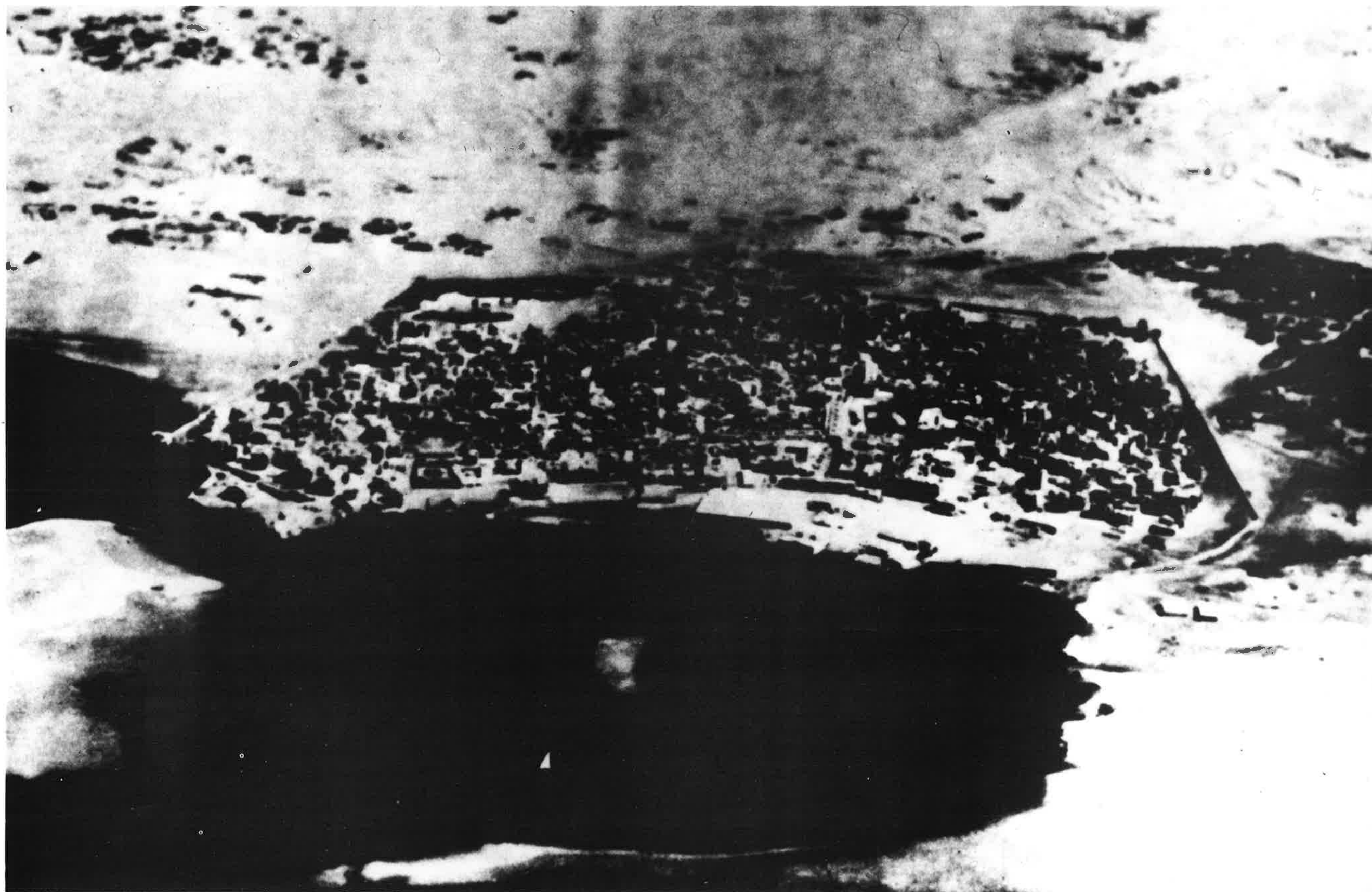
Aerial photograph of 'Old Jeddah' showing walls, circa 1930's
