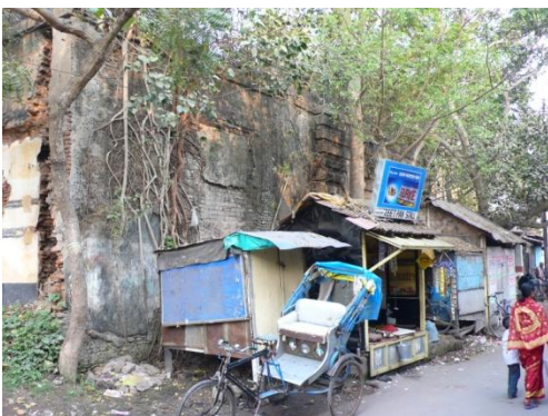
The southern gateway building of the compound obscured by vendor stalls
